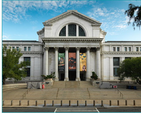
National Museum of Natural History Renovation 350,000 SF Site and stormwater
