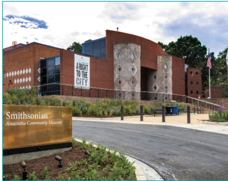
Anacostia Community Museum Center for African American Culture Renovation 28,000 SF
